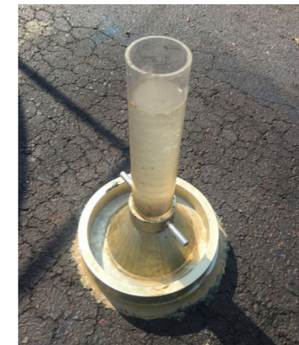
No water seepage into cracked seal.
