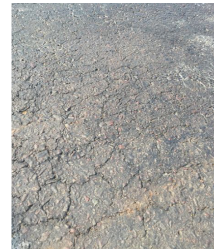
Area after Pavement seal has dried.
