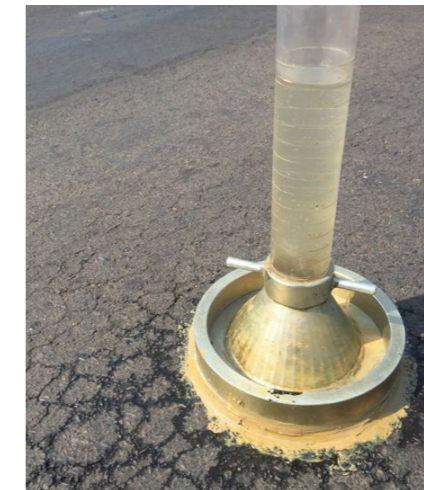
Water seepage into the layer finding its way through the cracked seal.
